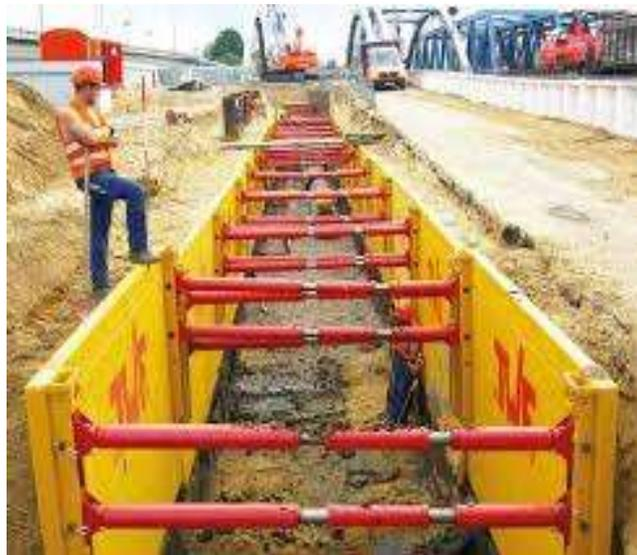
Figure 2. 22: Box Shoring System, (Source: Detailed Feasibility study)
